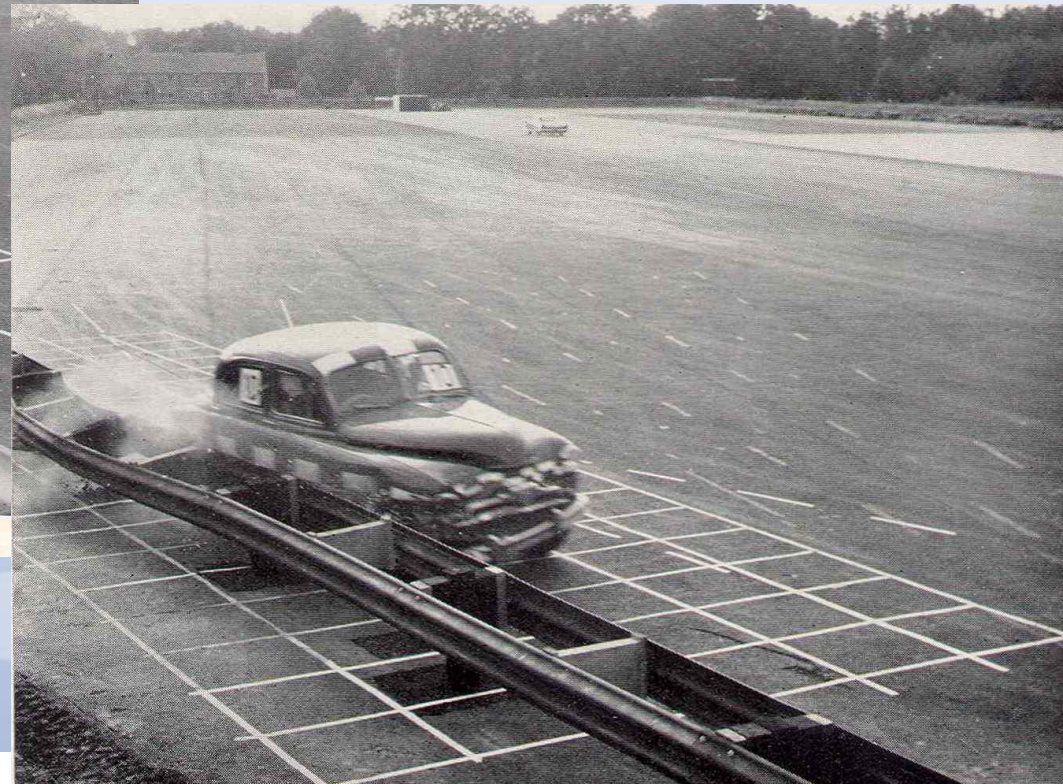
Impact with D.A.V. concrete guard rail at 46 mile/h and 20°
