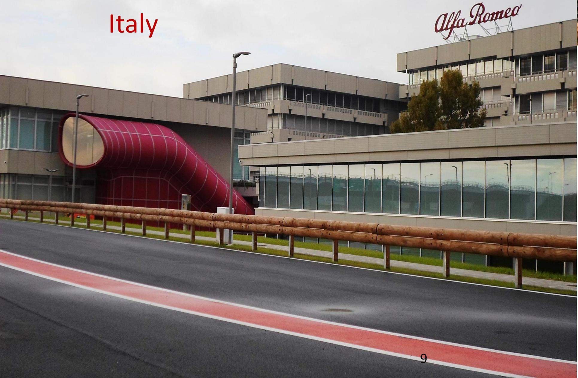
Mixed Wood & Steel Guardrails:
